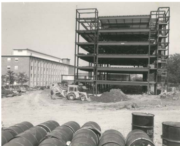
Seeley G. Mudd building under construction, circa October 1974
